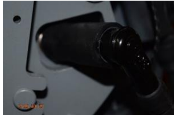
Fig (6) 2" Boot Cover installed
